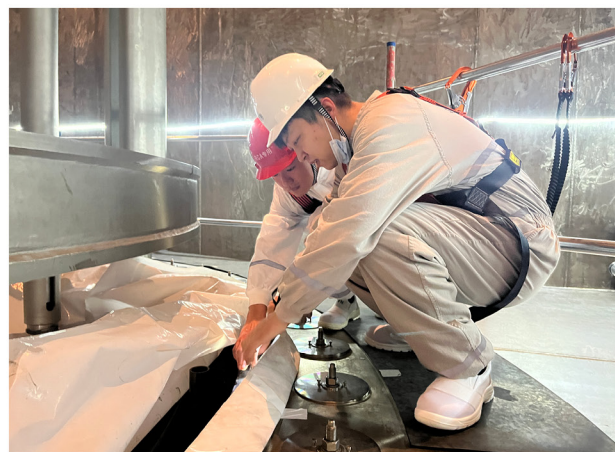
Figure 21. On-site Inspection on Uncovered Sealing Surface of Pressure Vessel for CAP1400 Demonstration Project
