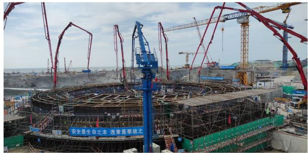
Figure 15. Concrete Pouring Site of Taipingling NPP Unit 1
