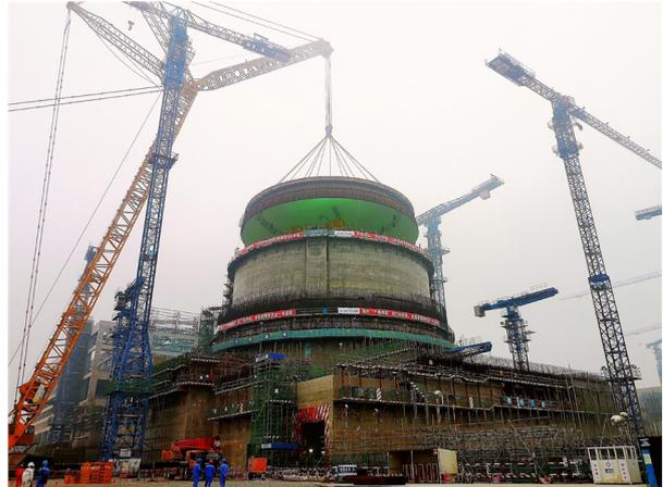
*Figure 9. Dome Hoisting of Fangchenggang NPP Unit 4*
