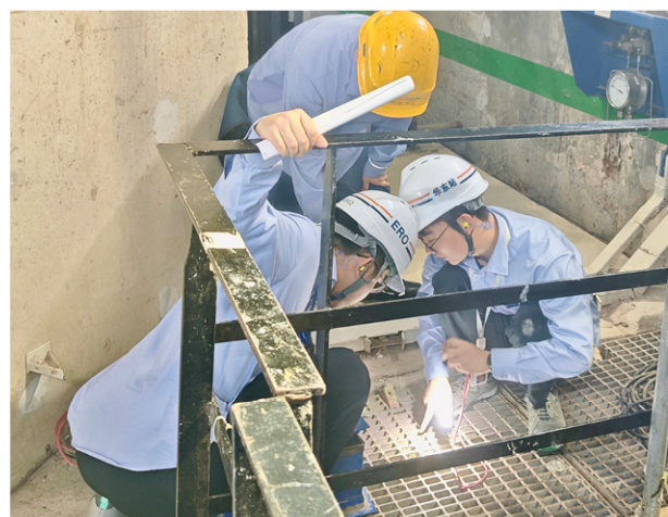
Figure 12. Regulatory Inspection on Combined Pump House at Ningde NPP
