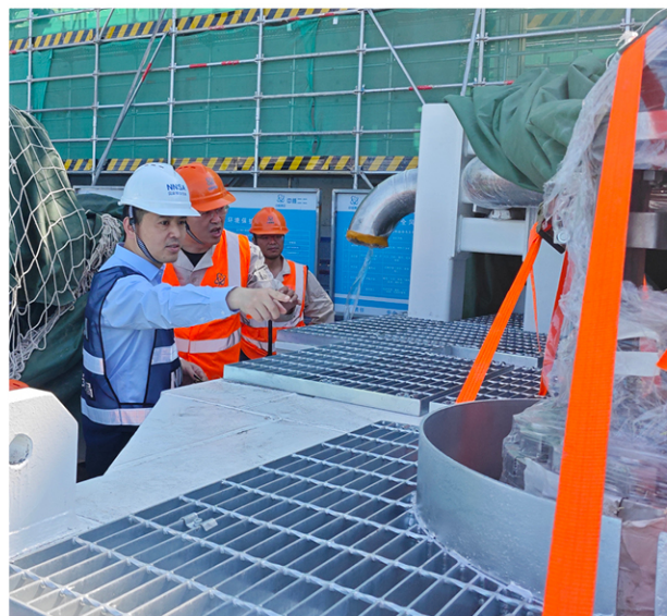
Figure 27. Regulatory Inspection on the Effectiveness of the Civil Construction Quality Assurance of Xudapu NPP Unit 2
