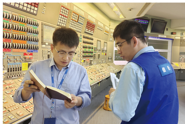
Figure 6. Regulatory Inspection in the Main Control Room of Qinshan Phase III NPP
