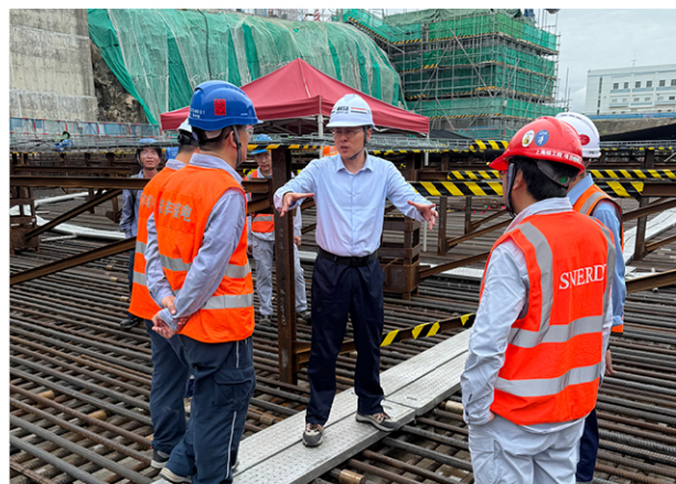
Figure 28. Inspection on the Base Plate Bar Binding of Lufeng NPP Unit 2
