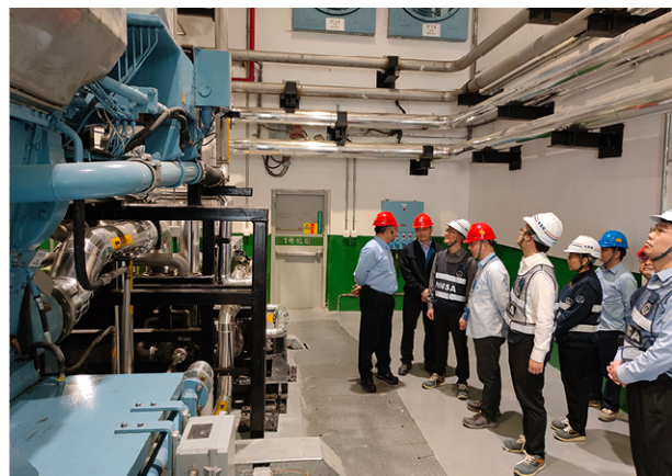
Figure 4. Regulatory Inspection on Renovation of Emergency Diesel Engine at Qinshan NPP
