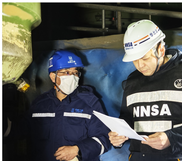
Figure 10. Regulatory Inspection on Main Pipeline Welding at Tianwan NPP Unit 8
