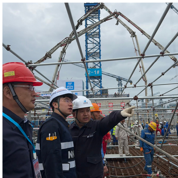
Figure 22. Regulatory Inspection on FCD of Unit 2, Phase I Expansion Project of Shidao Bay NPP
