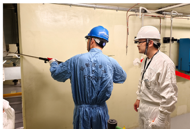
Figure 20. Regulatory Inspection on Nuclear Auxiliary Building at Fangchenggang NPP
