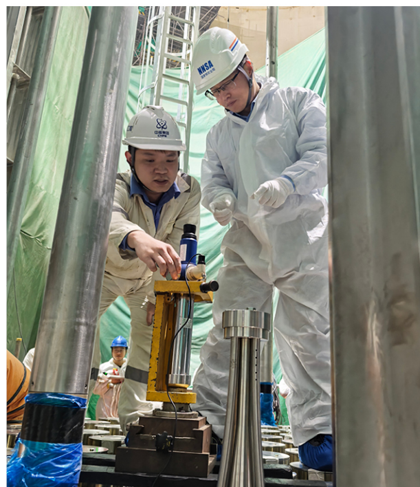
Figure 19. Regulatory Inspection on Reactor Internals of Changjiang NPP Unit 4
