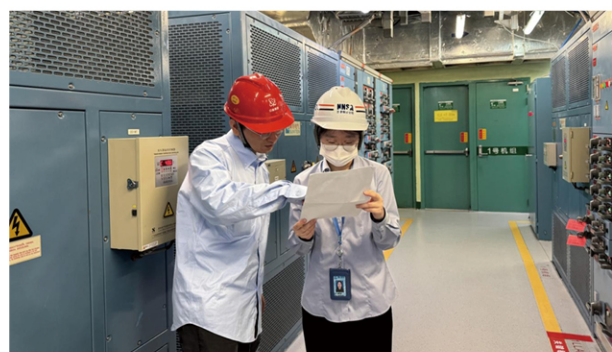
Figure 7. Regulatory Inspection on Electrical Building at Fangjiashan NPP
