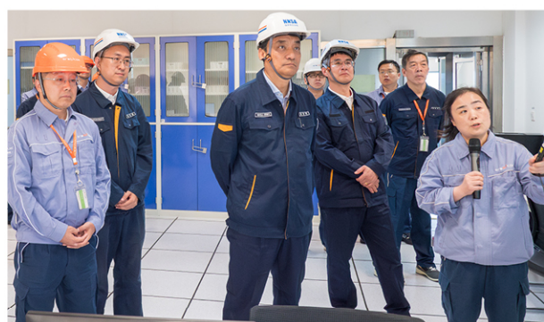
Figure 17. DONG Baotong, Vice Minister of Ecology and Environment and Administrator of the National Nuclear Safety Administration, conducted filed investigations of the central station of the environmental monitoring system at Taishan NPP
