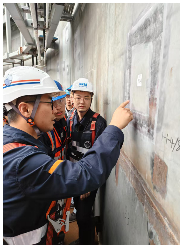
Figure 29. Regulatory Inspection on the CV Attachment Plate Cutting and Rewelding of Lianjiang NPP
