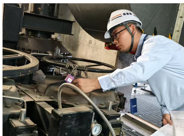
Figure 13. Regulatory Inspection on Main Steam Isolation Valve Room at Fuqing NPP
