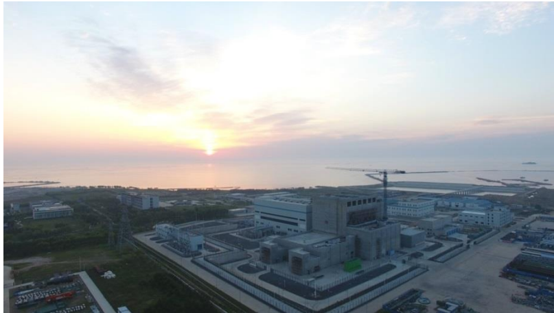
Figure 9. HTGR Demonstration Project Construction Site
