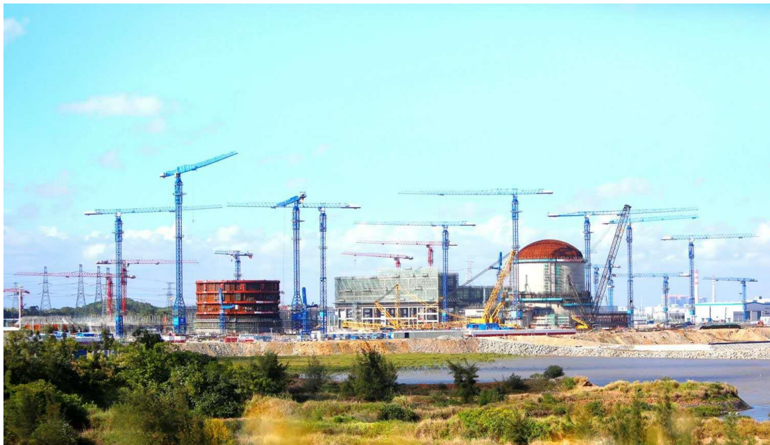
Figure 8. Construction Site of Fangchenggang NPP Unit 3 and Unit 4
