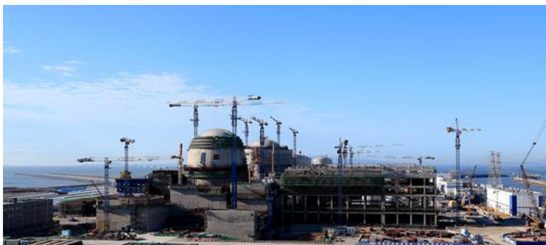
Figure 5. Construction Scene of Fuqing Nuclear Power Plant
