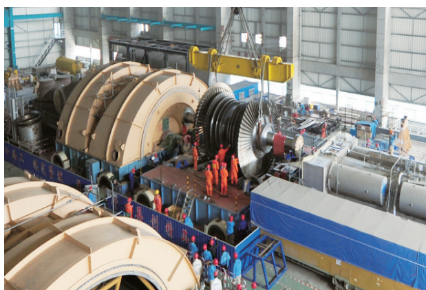
Steam Turbine Installation of Ningde Unit 2
