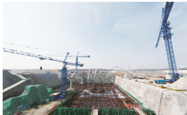
Concrete Pouring of NI Baseplate 2m Floor
