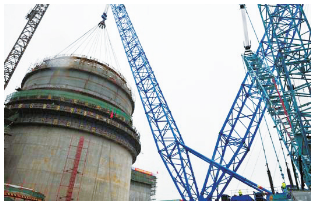
Hoisting in Position for the Containment Top Head of Unit 1
