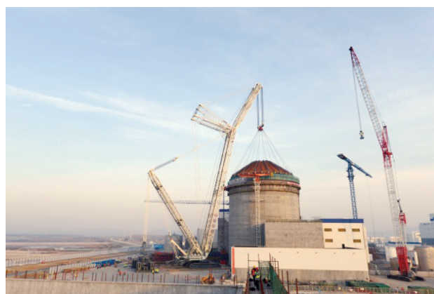
The Steel Containment Dome of Shield Building Installed in Place of Haiyang NPP Unit 1
