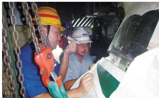
Primary Pipe Welding of Changjiang NPP Unit 1
