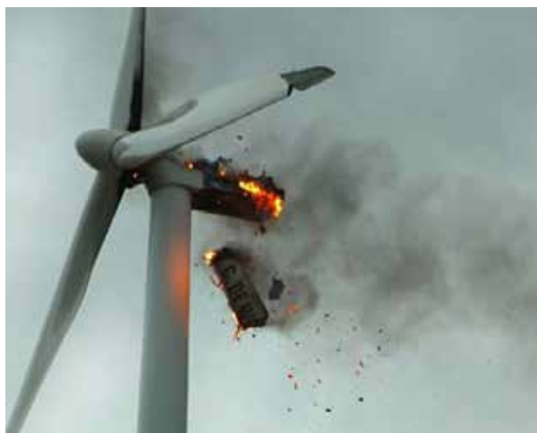
图1-4-8 风力发电机烧毁
