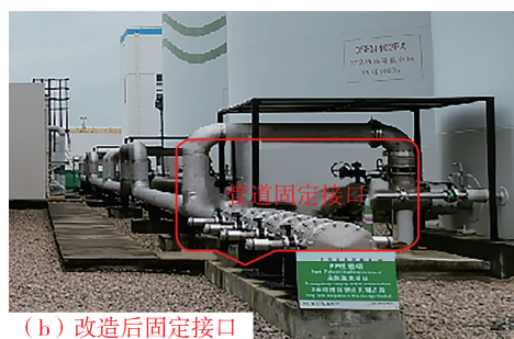
图 2 SED/SER 系统水箱 DN350 管道固化前后比较 Fig.2 Comparison of SED/SER DN350 pipeline before and after curing
