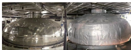
图3 蒸发器表面传统硬质保温盒和穿戴式软质保温 Fig.3 Traditional hard insulation box and wearable soft insulation for evaporator surface
