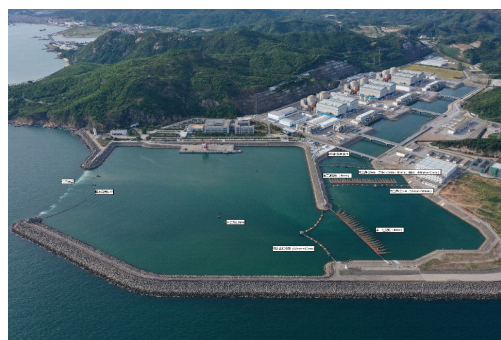
图1 阳江核电厂冷源拦截设施布置总体图 Fig.1 General layout of cold source interception facilities of Yangjiang nuclear power plant
