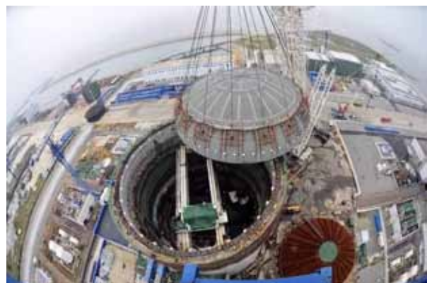
Top Head Hoisting of the Steel Containment of Haiyang NPP unit 2
