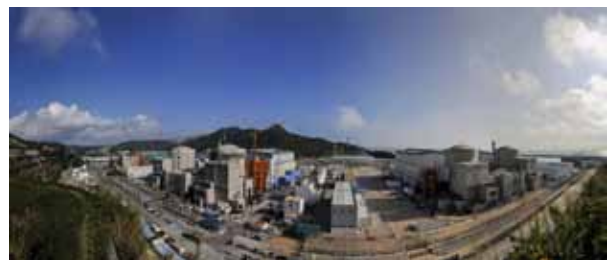
Overall View of Yangjiang NPP Unit 1 to Unit 6
