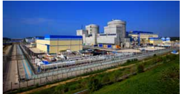
View of the Nuclear Island of Changjiang NPP Unit 1 and Unit 2
